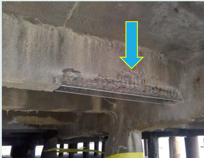
Music Pier Substructure Repairs - $ 517K
